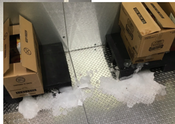
Figure 2 - Floor Before with Digital Controller
