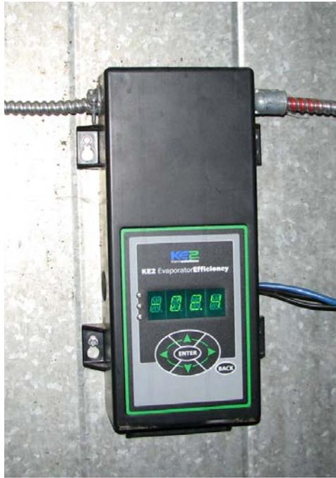
The controller, installed outside of the refrigerated space, displays the temperature in tenths of a degree, and is visible without entering the freezer.
